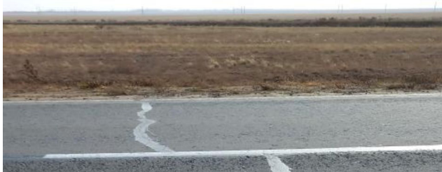
Fig. 4. Typical result of the road geometry's acquisition.
